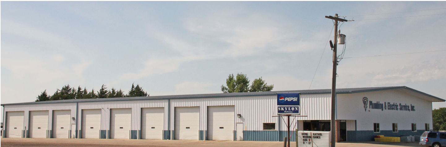
Plumbing and Electric Service Inc.
