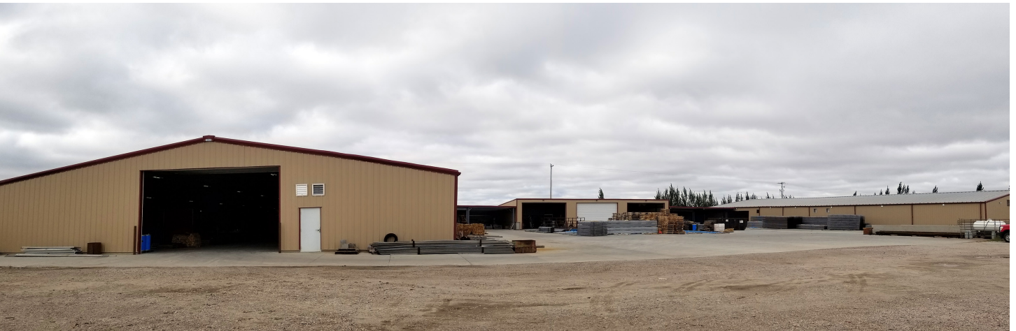
Northeast Pipe and Panel Hartington
