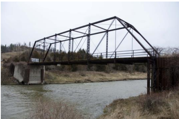
Photograph 6.4 County Line Bridge Source: Nebraska Historical Society
