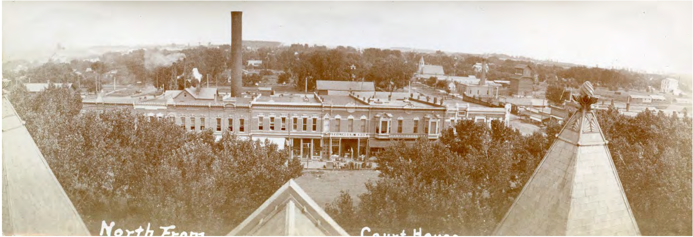
Buildings 8-16 (original 16 building) can see original 2 nd story windows better.
