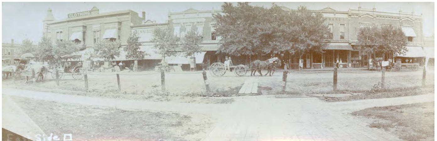
Buildings 34-42, 1897, can see some original upper story windows.
