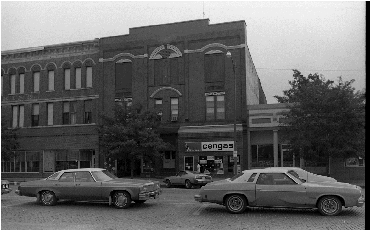
Focus on building 57, opera house, 1980
